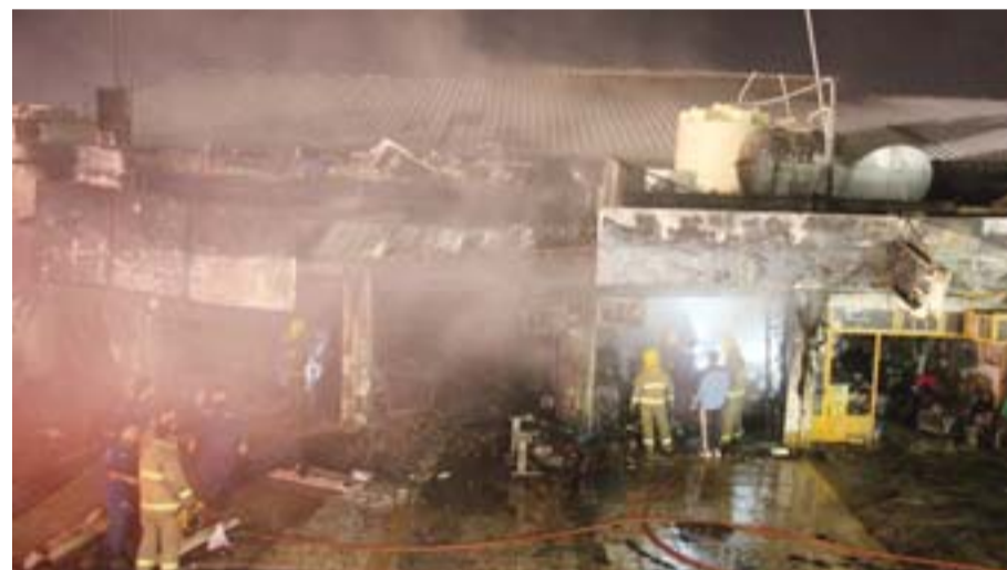
KUWAIT: Firefighters battle a blaze at car repair shops in Shuwaikh Industrial.
