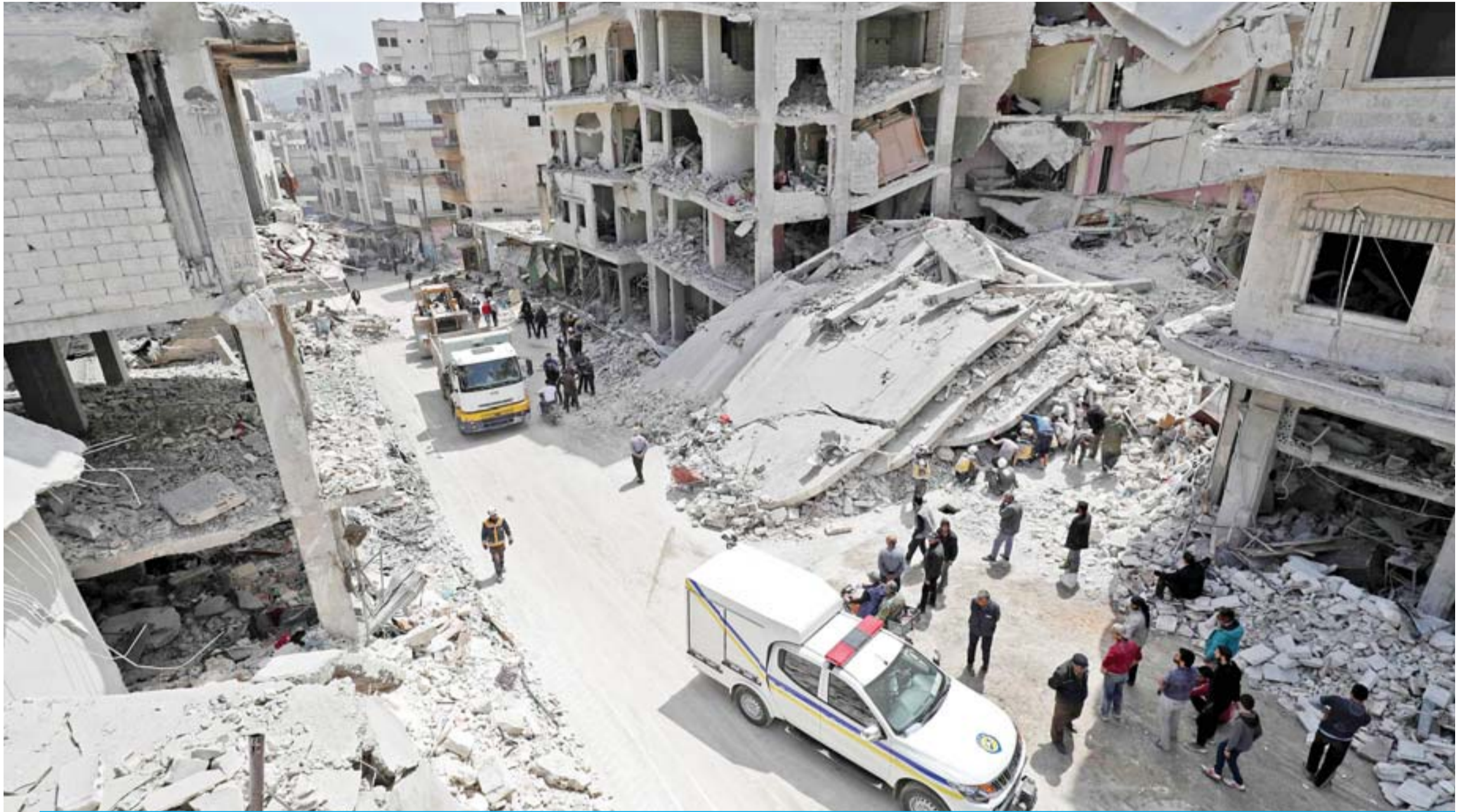
JISR ASH SHUGHUR, Syria: People watch as members of the Syrian Civil Defense, also known as the 'White Helmets', search the rubble of a collapsed building following an explosion in the town of Jisr al-Shughur, in the west of the mostly rebel-held Syrian province of Idlib. — AFP
