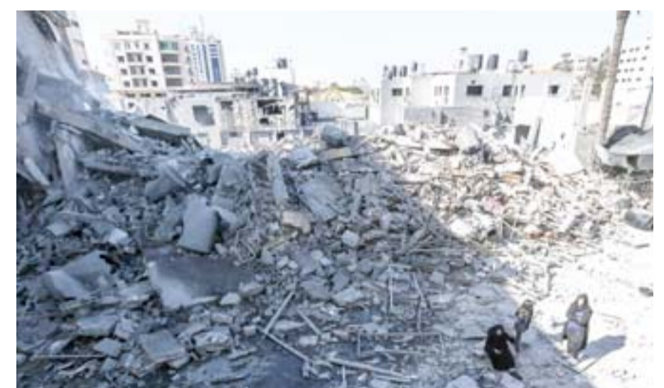
GAZA: Palestinians gather next to the rubble of a building in Gaza City, after Israeli air strikes hit dozens of sites across the Strip overnight in response to rocket fire from the Palestinian enclave. — AFP
