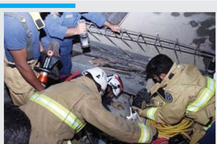
KUWAIT: Fire and rescue personnel try to free workers who were trapped after the roof of an under-construction mosque collapsed yesterday.
