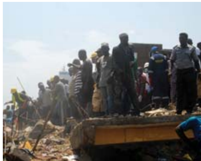
LAGOS: Emergency and rescue personnel are seen at the site of a building which collapsed in Lagos.—AFP
