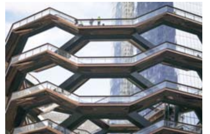
Workers walk on 'The Vessel' in the Hudson Yards development on the West Side of Midtown Manhattan.
