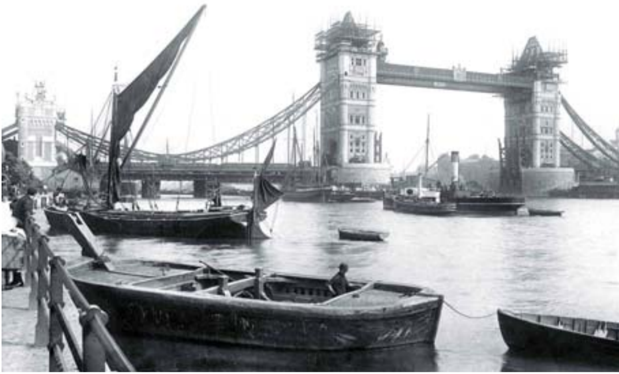
A handout archive picture taken in 1893 shows Tower Bridge under construction in London. — AFP photos
