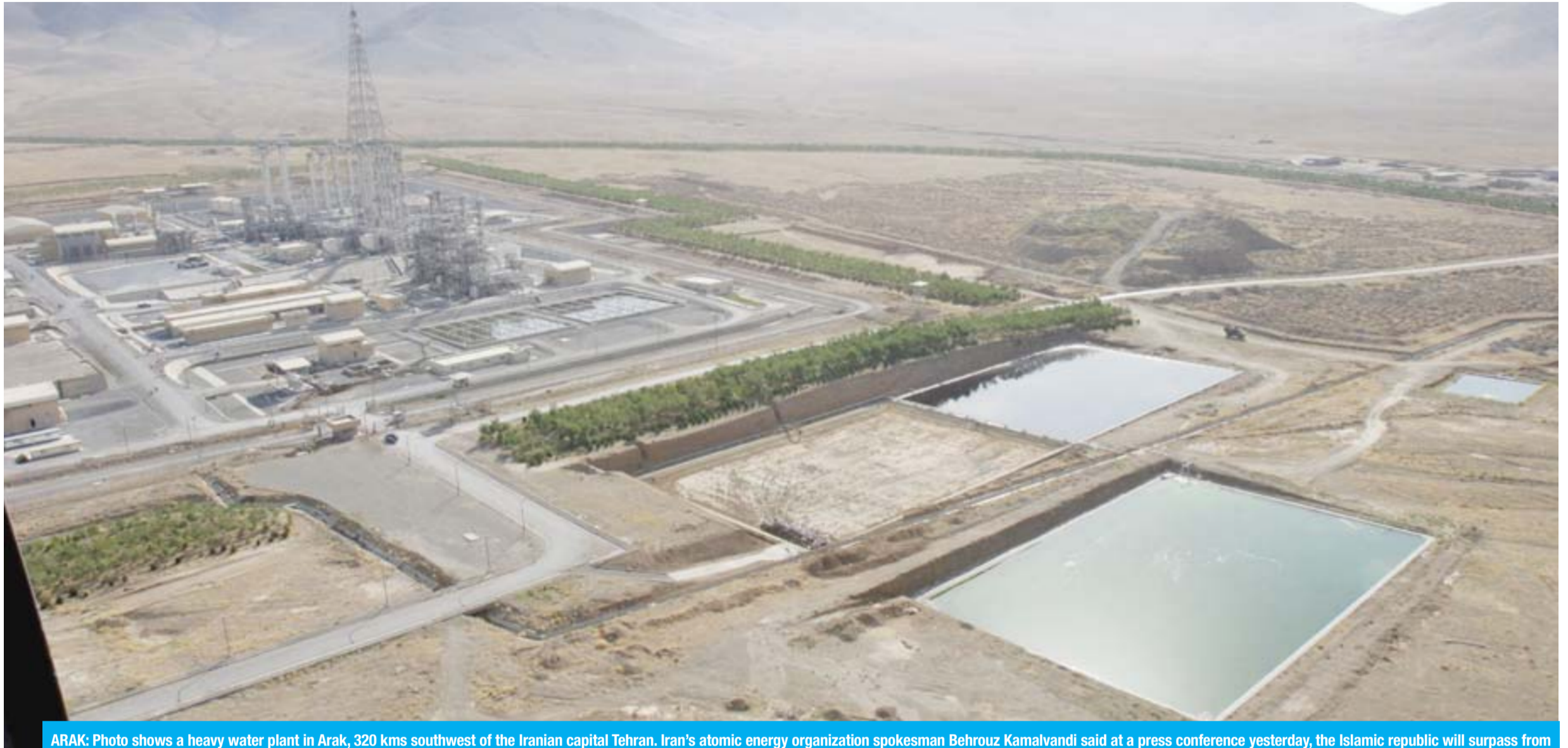
ARAK: Photo shows a heavy water plant in Arak, 320 kms southwest of the Iranian capital Tehran. Iran's atomic energy organization spokesman Behrouz Kamalvandi said at a press conference yesterday, the Islamic republic will surpass from June 27 its uranium stockpile limit set under the nuclear deal with world powers, turning up the pressure after the US walked away from the landmark pact last year. — AFP
