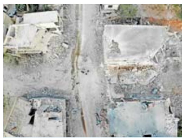
IHSIM: Photo shows damaged and destroyed buildings in the town of Ihsim, in Syria's Idlib region. — AFP
