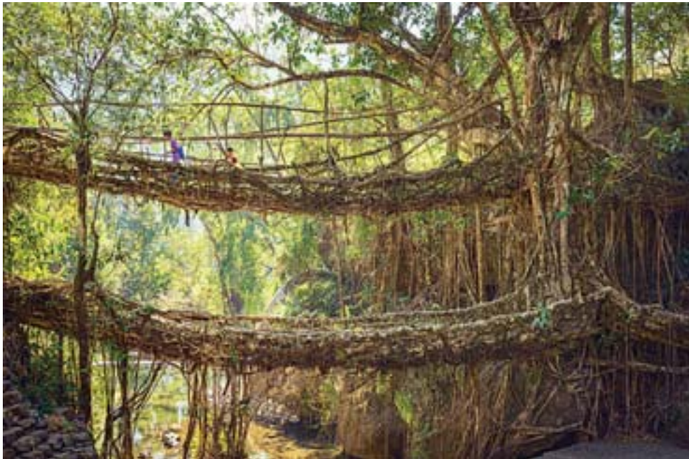
The living root bridges of Meghalaya have become a poster child for the sense of mysticism surrounding India's remote Northeast
