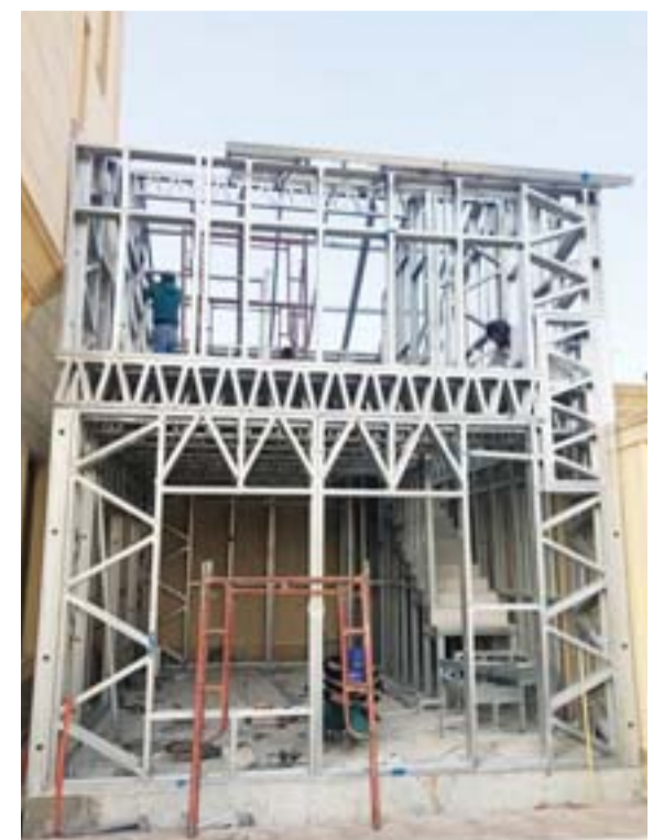
Construction workers install galvanized steel at a house in Kuwait.
