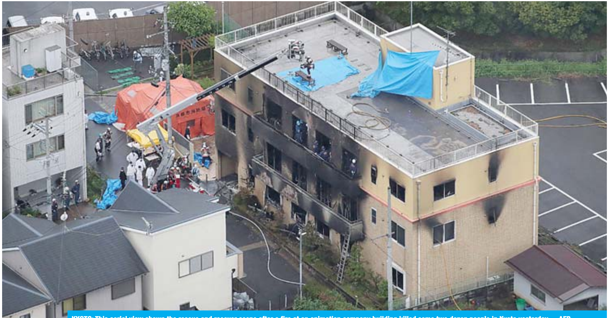
KYOTO: This aerial view shows the rescue and recover scene after a fire at an animation company building killed some two dozen people in Kyoto yesterday. —AFP
