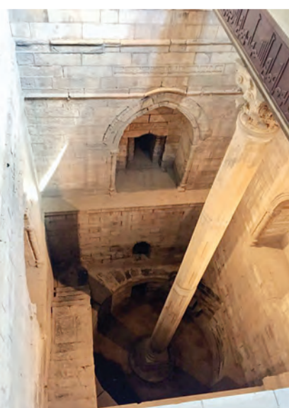
A Marble column for measuring water level.
