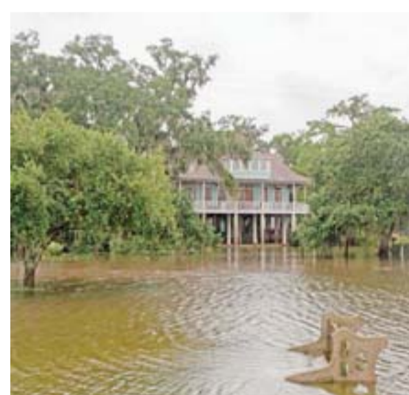
MANDEVILLE: Flood waters cover a neighborhood street after Tropical Storm Barry passed through in Mandeville, Louisiana. — AFP
