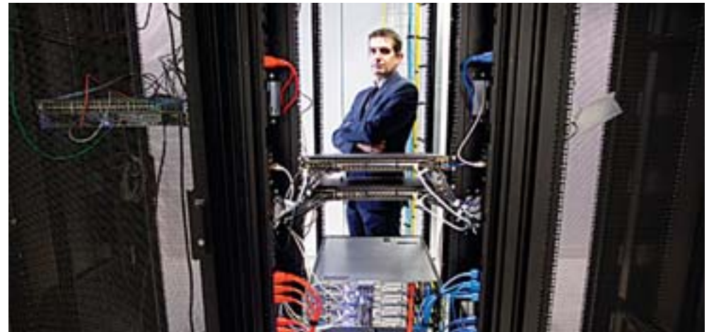
DUBLIN: Commercial Director, Brian Roe poses for a photograph beside the cabinets inside Servecentric Data Centre on the outskirts of Dublin. —AFP
