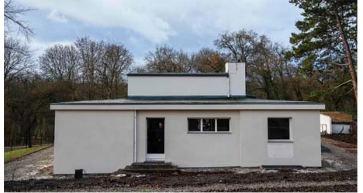
View of the "Haus am Horn", designed by Georg Muche for the major Bauhaus Exhibition of 1923.
