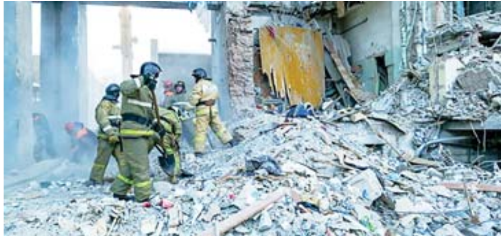
MOSCOW: This handout photograph shows rescuers taking part in a search operation three days after a gas explosion rocked a residential building in Russia's Urals city of Magnitogorsk.—AFP
