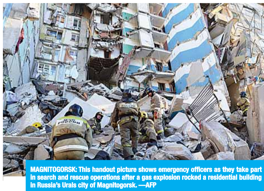
MAGNITOGORSK: This handout picture shows emergency officers as they take part in search and rescue operations after a gas explosion rocked a residential building in Russia's Urals city of Magnitogorsk. —AFP
