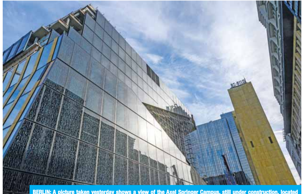
BERLIN: A picture taken yesterday shows a view of the Axel Springer Campus, still under construction, located just opposite German media giant Axel Springer's current headquarters in Berlin. — AFP
