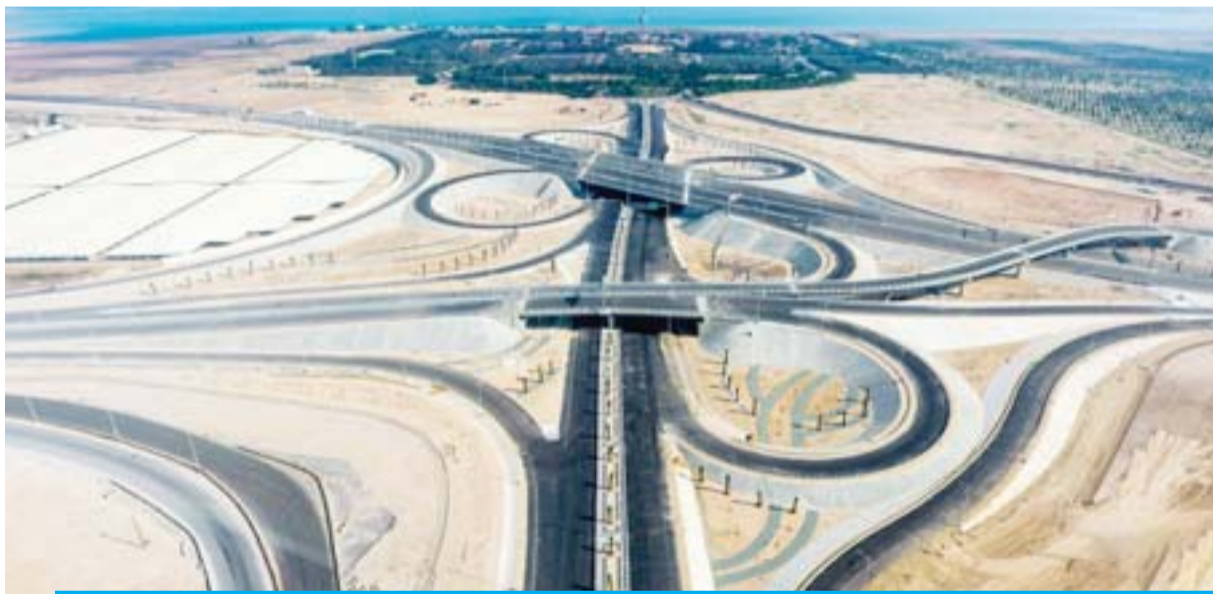
An aerial view of the Sheikh Jaber Causeway's intersections.
