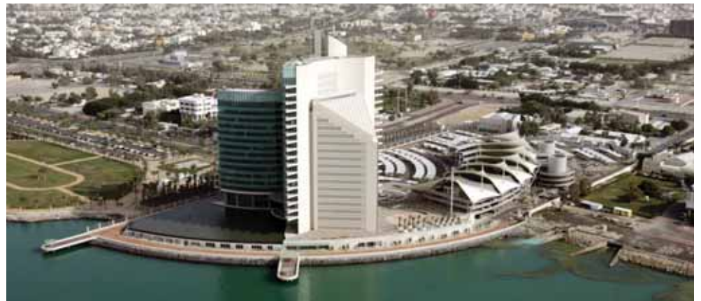
KUWAIT: An archive photo showing Kuwait Petroleum Corporation's building in Kuwait City. — KUNA
