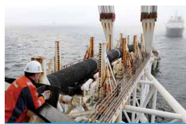
In this file photo, an employee of the Allseas offshore service company works on the ship "Audacia", from where parts of the Nord Stream 2 pipeline are laid in the Baltic Sea off the coast of Laage, northeastern Germany. —AFP
