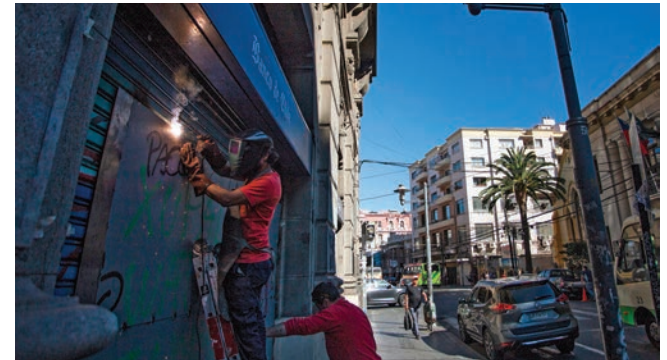
Men work on the security of a bank's shutter.
