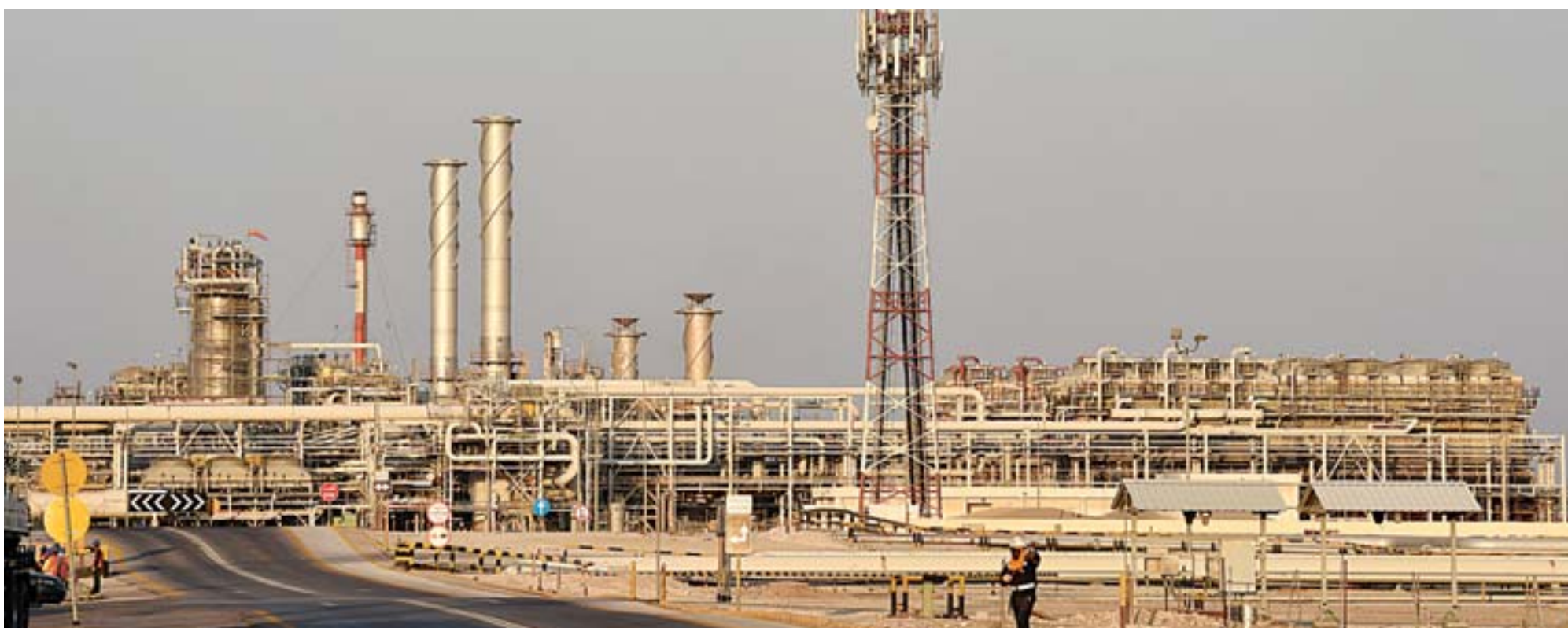
ABQAIQ: Photo shows a general view of Saudi Aramco's Abqaiq oil processing plant. Saudi Aramco's shares soared on their debut on the domestic stock exchange - becoming the world's biggest listed company worth $1.88 trillion after a record-breaking IPO. —AFP
