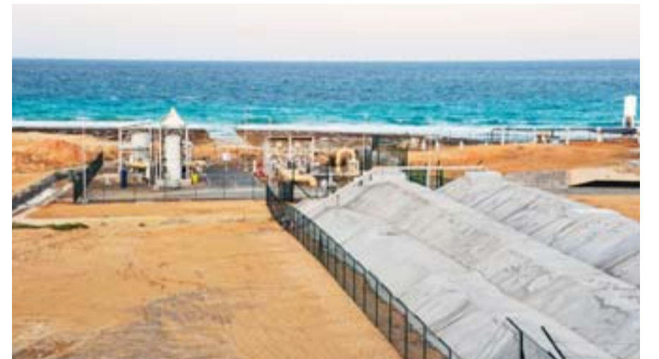
AS SUR, Oman: A view of a desalination plant in the Omani port city of Sur, south of the capital Muscat. — AFP
