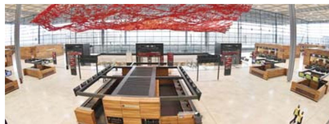
BRANDENBURG: Photo shows the entry hall to the Berlin-Brandenburg Willy-Brandt international Airport in Schoenefeld, near Berlin. — AFP
