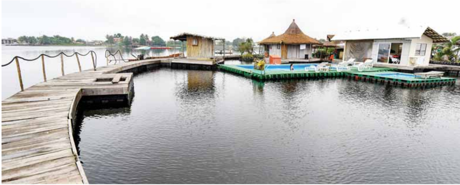
View of the resort on an artificial island made with around 700,000 recycled plastic waste collected in the surrounding area. —AFP photos
