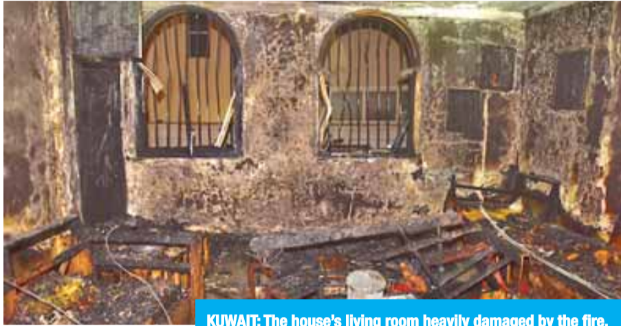
KUWAIT: The house's living room heavily damaged by the fire.
