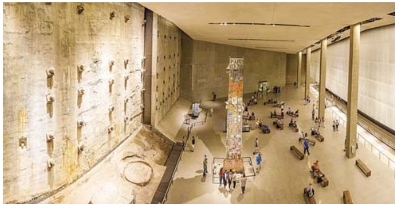
The subterranean concrete wall in the National September 11 Memorial Museum, New York City.
