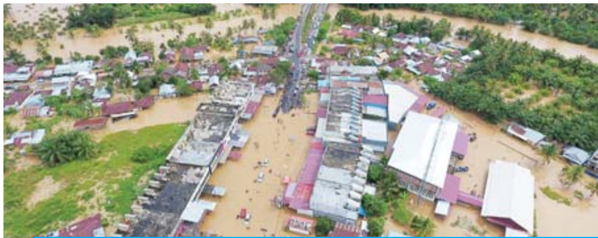
BENGKULU: This aerial picture shows a general view of submerged buildings after heavy rain caused flooding in Bengkulu on the Indonesian island of Sumatra. — AFP
