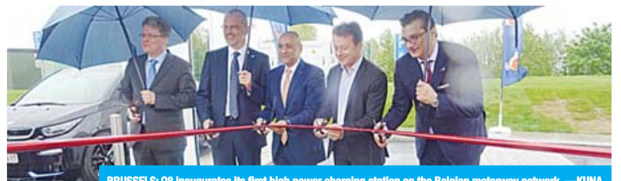
BRUSSELS: Q8 Inaugurates its first high power charging station on the Belgian motorway network. —KUNA
