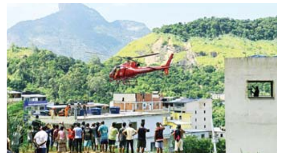
RIO DE JANEIRO: People watch a rescue helicopter as it flies away carrying an injured person after two buildings collapsed in Muzema, Rio de Janeiro. — AFP
