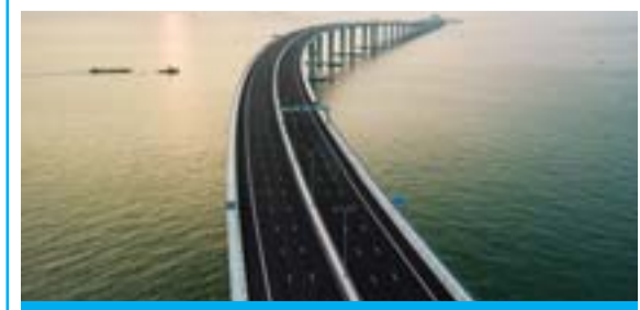
HONG KONG: An aerial view taken on Monday shows a section of the Hong Kong-Zhuhai-Macau Bridge (HKZM). — AFP
