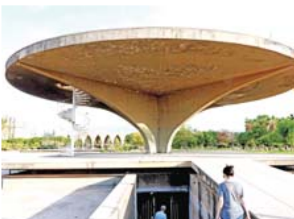
A view of the concrete helicopter platform at the grounds of the Tripoli International Fair, close to the seafront of the northern Lebanese port city. — AFP photos
