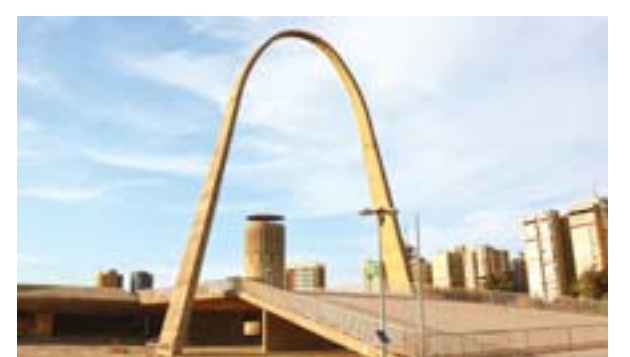
A view of the thin concrete arch at the grounds of the Tripoli International Fair.
