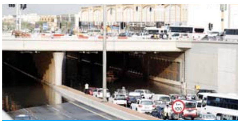
DOHA: Motorists drive through a flooded tunnel in the Qatari capital following heavy rainfall on Saturday. — AFP
