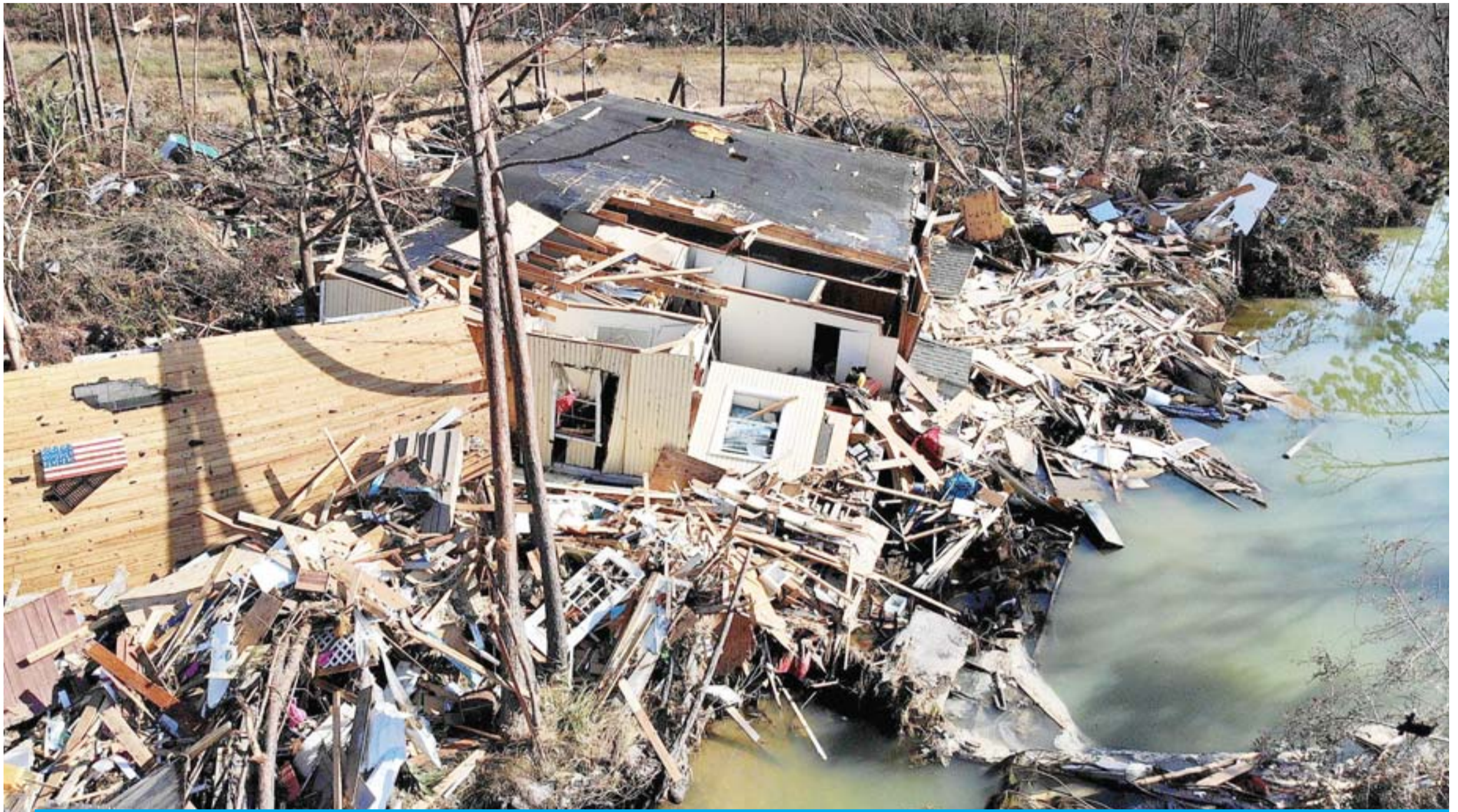
FLORIDA: A destroyed house sits in debris and rubble in the aftermath of Hurricane Michael in Mexico Beach, Florida. The hurricane hit on October 10 along the Florida Panhandle as a category 4 storm causing massive damage and claimed the lives of more than a dozen people. —AFP
