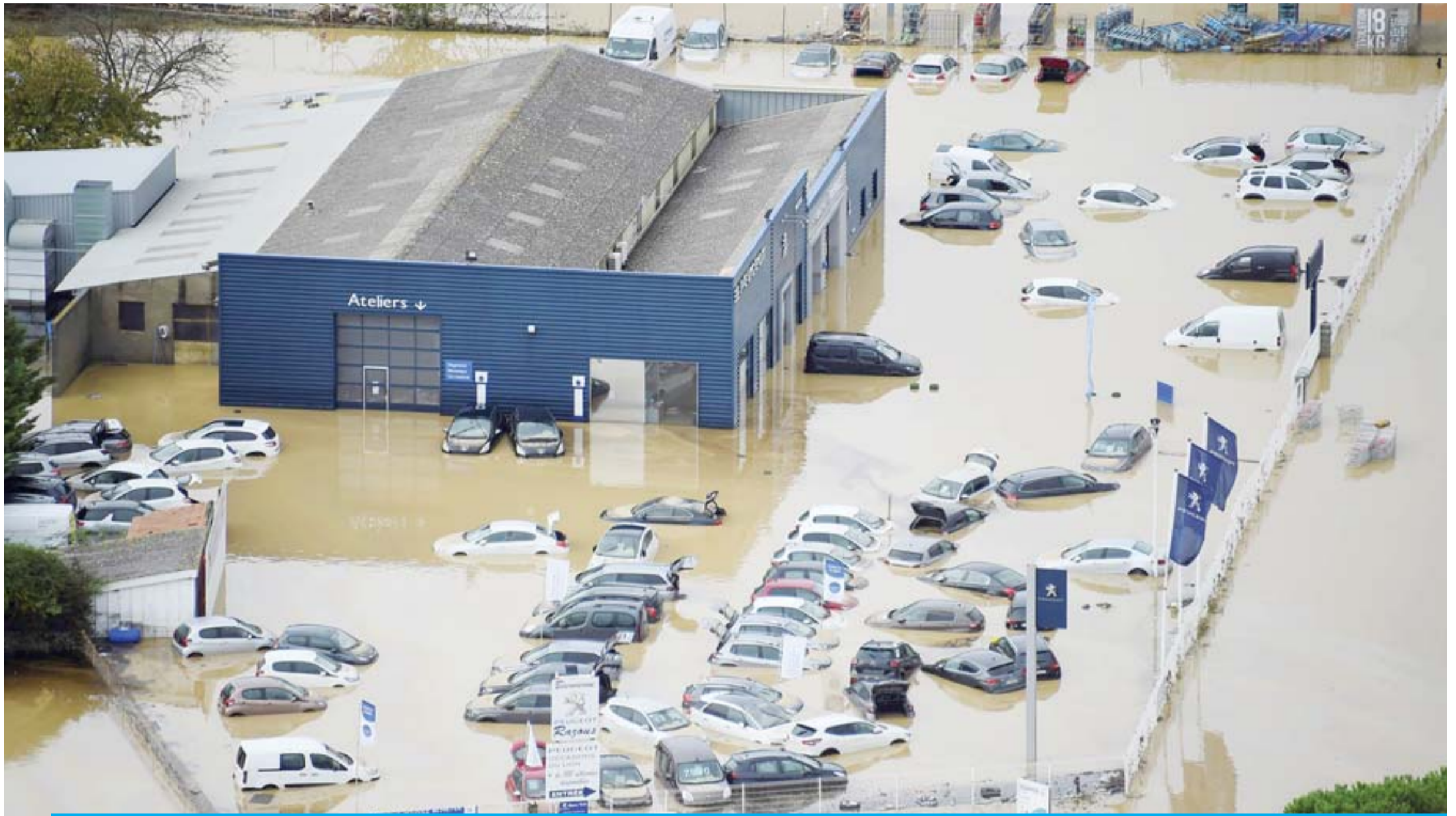
VILLEGAILHENC: An aerial view shows a flooded Peugeot car maker garage in the city of Villegailhenc, near Carcassonne, southern France, following heavy rains that saw rivers bursting banks. — AFP
