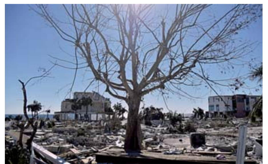
MEXICO BEACH: View of the damage caused by Hurricane Michael in Mexico Beach, Florida, four days after Hurricane Michael hit the area. —AFP
