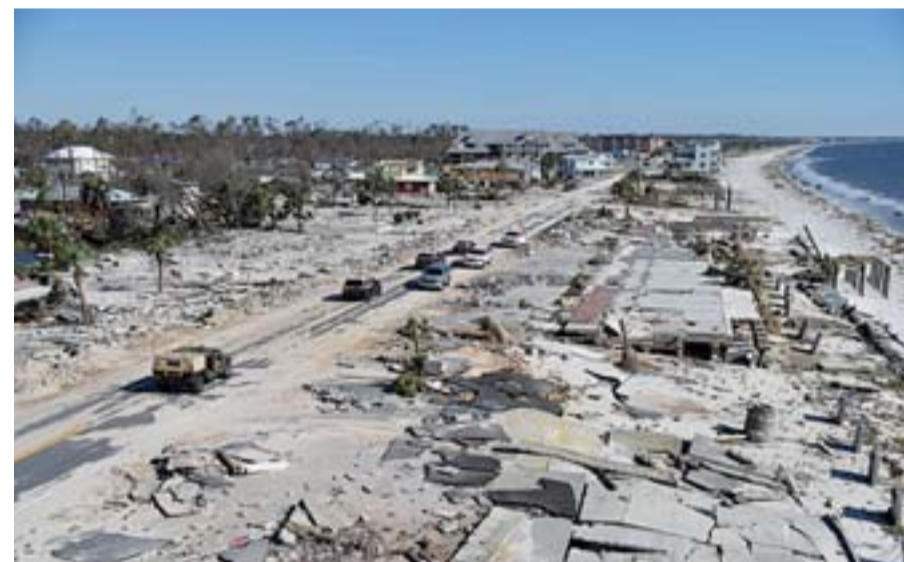
MEXICO BEACH: View of the damaged caused by Hurricane Michael in Mexico Beach, Florida. —AFP
