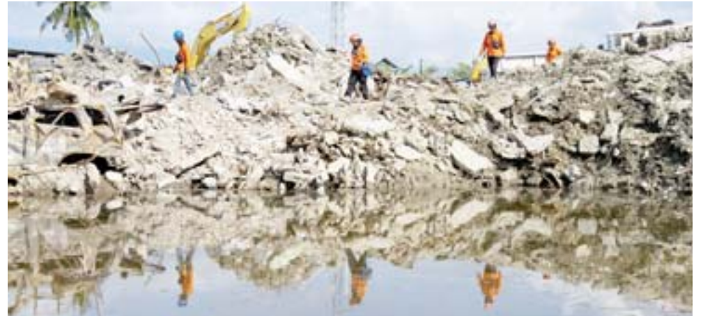
PALU: Indonesian search and rescue personnel work on the final day of recovery operations at soil liquefaction-hit Balaroa village in Palu yesterday, following the September 28 earthquake and tsunami that hit the area. — AFP
