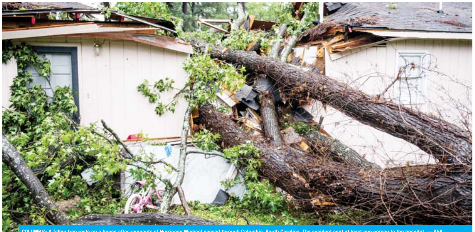
COLUMBIA: A fallen tree rests on a house after remnants of Hurricane Michael passed through Columbia, South Carolina. The accident sent at least one person to the hospital. — AFP
