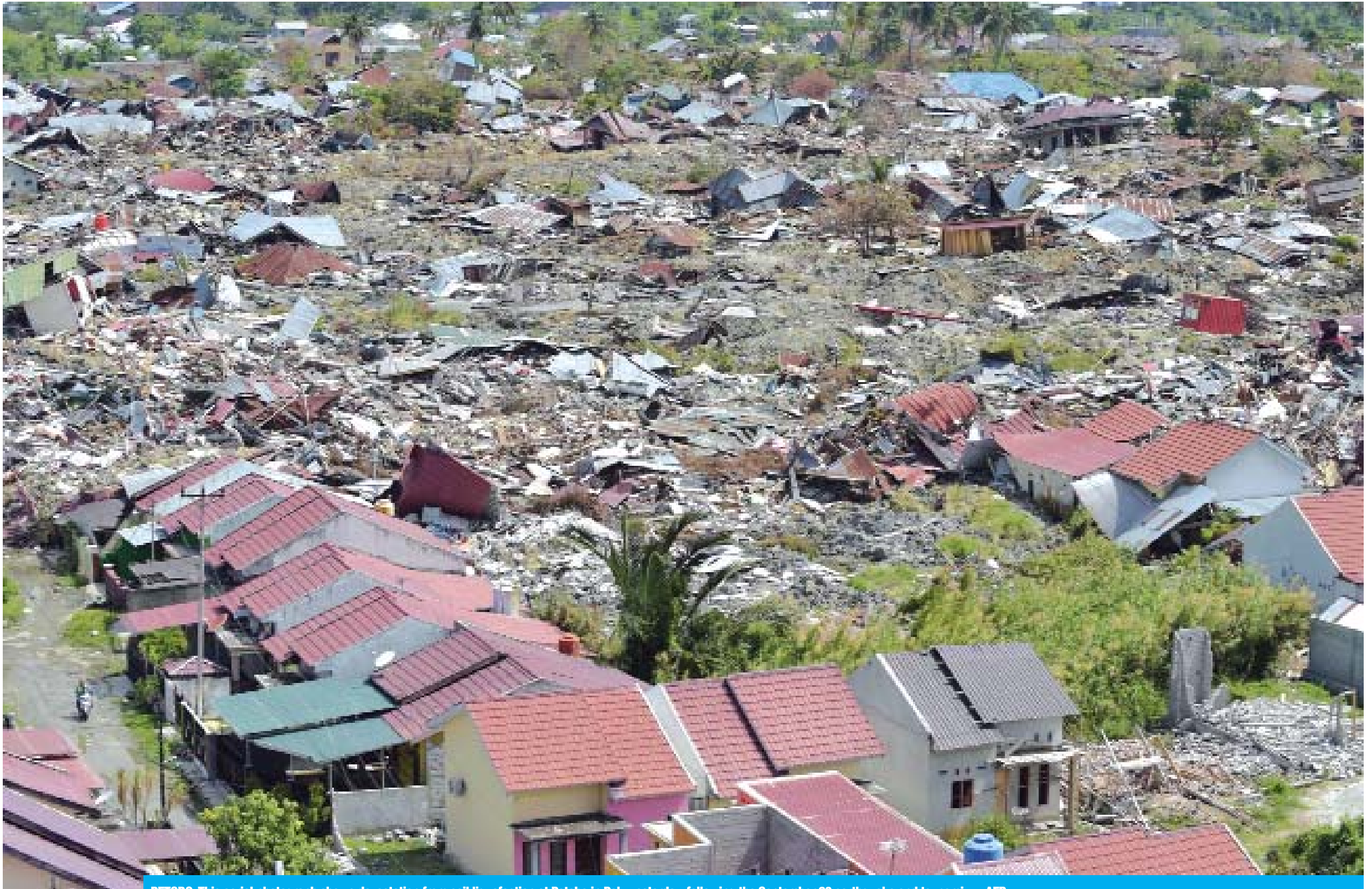
PETOBO: This aerial photograph shows devastation from soil liquefaction at Petobo in Palu yesterday, following the September 28 earthquake and tsunami. — AFP
