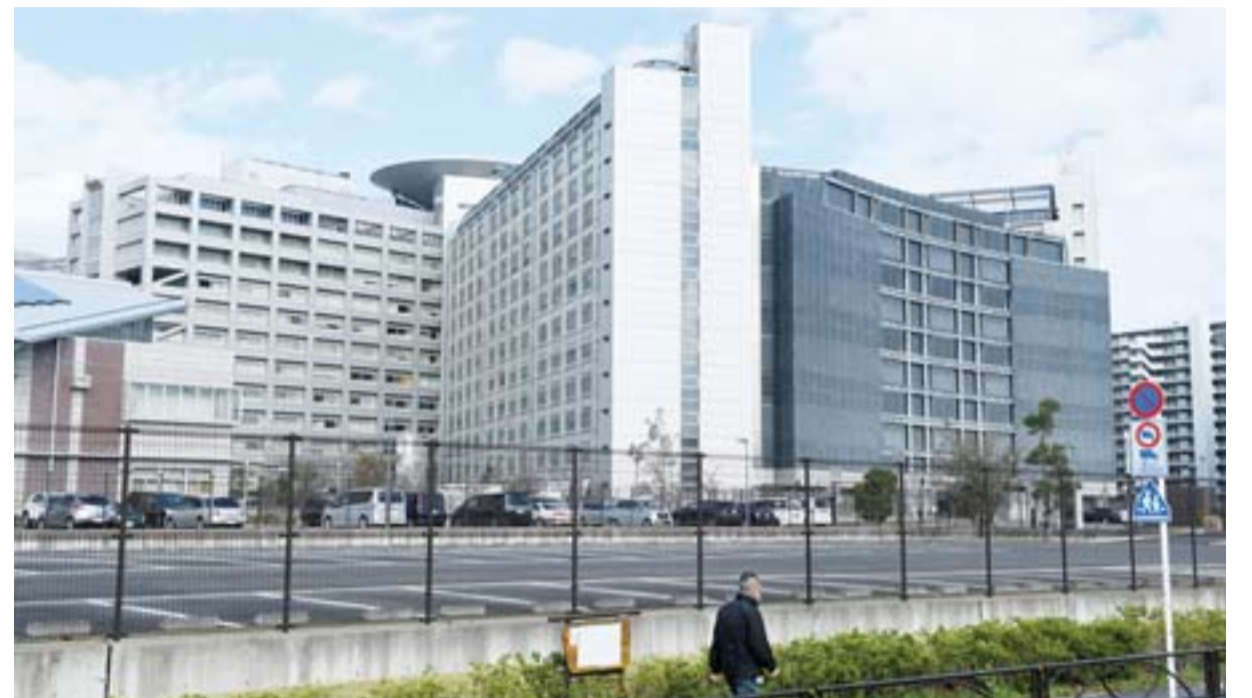
TOKYO: This general view shows the Tokyo Detention House in Katsushika. Sources told AFP on November 20 that Carlos Ghosn, one of the world's most influential executives, was being held at the detention center in the capital belonging to Tokyo prosecutors following his arrest the day before. — AFP
