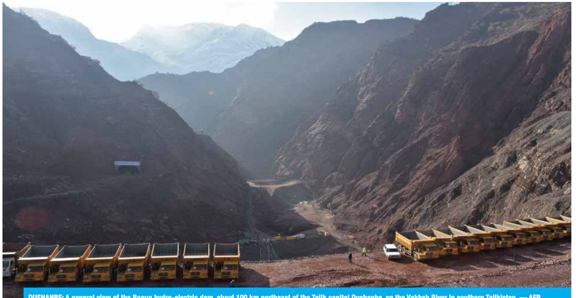
DUSHANBE: A general view of the Rogun hydro-electric dam, about 100 km northeast of the Tajik capital Dushanbe, on the Vakhsh River in southern Tajikistan. — AFP
