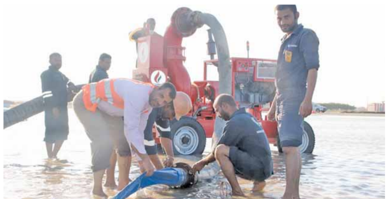
Workers drain rainwater at the airport.
