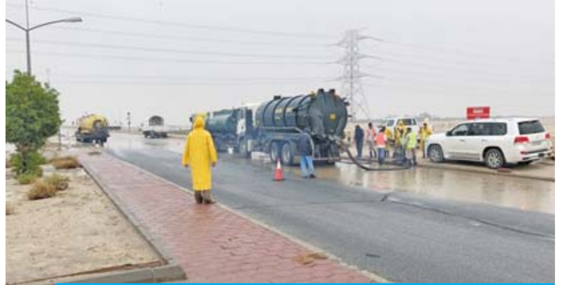
Public Works Ministry workers drain rainwater.
