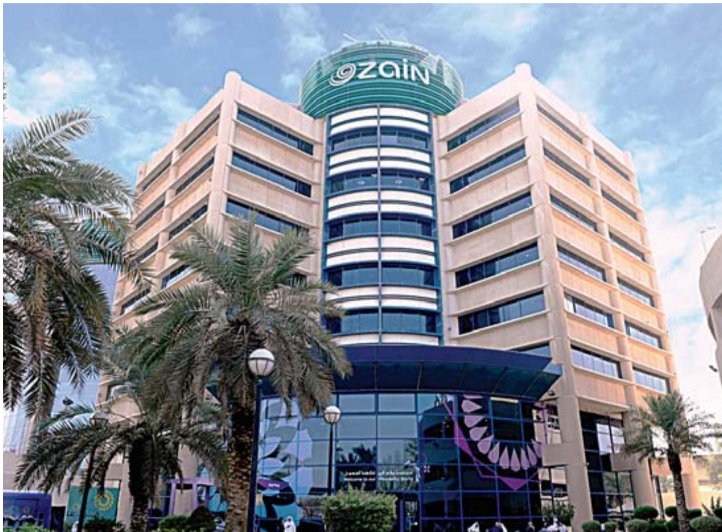
Zain's main HQ building
