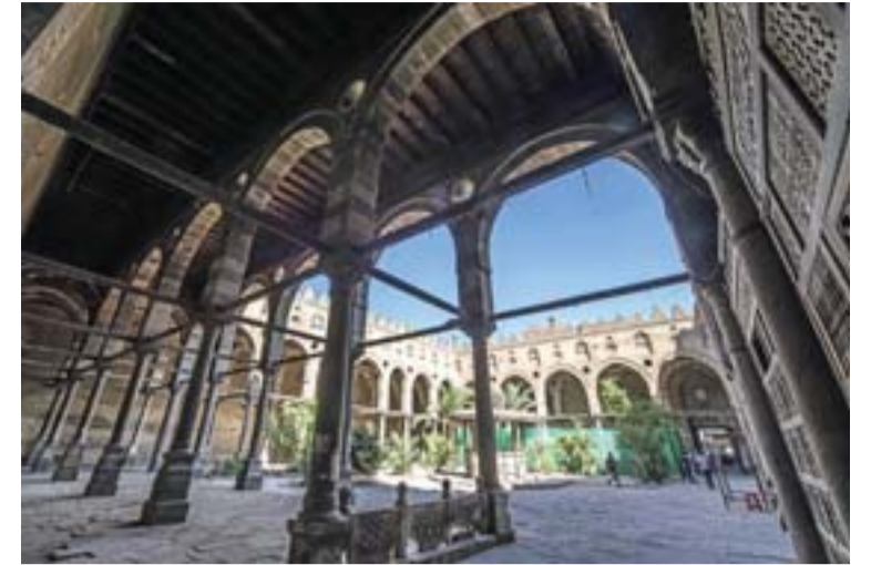
A picture shows the 14th century al-Maridani mosque at al-Darb al-Ahmar area in the capital Cairo, as it undergoes renovation works.
