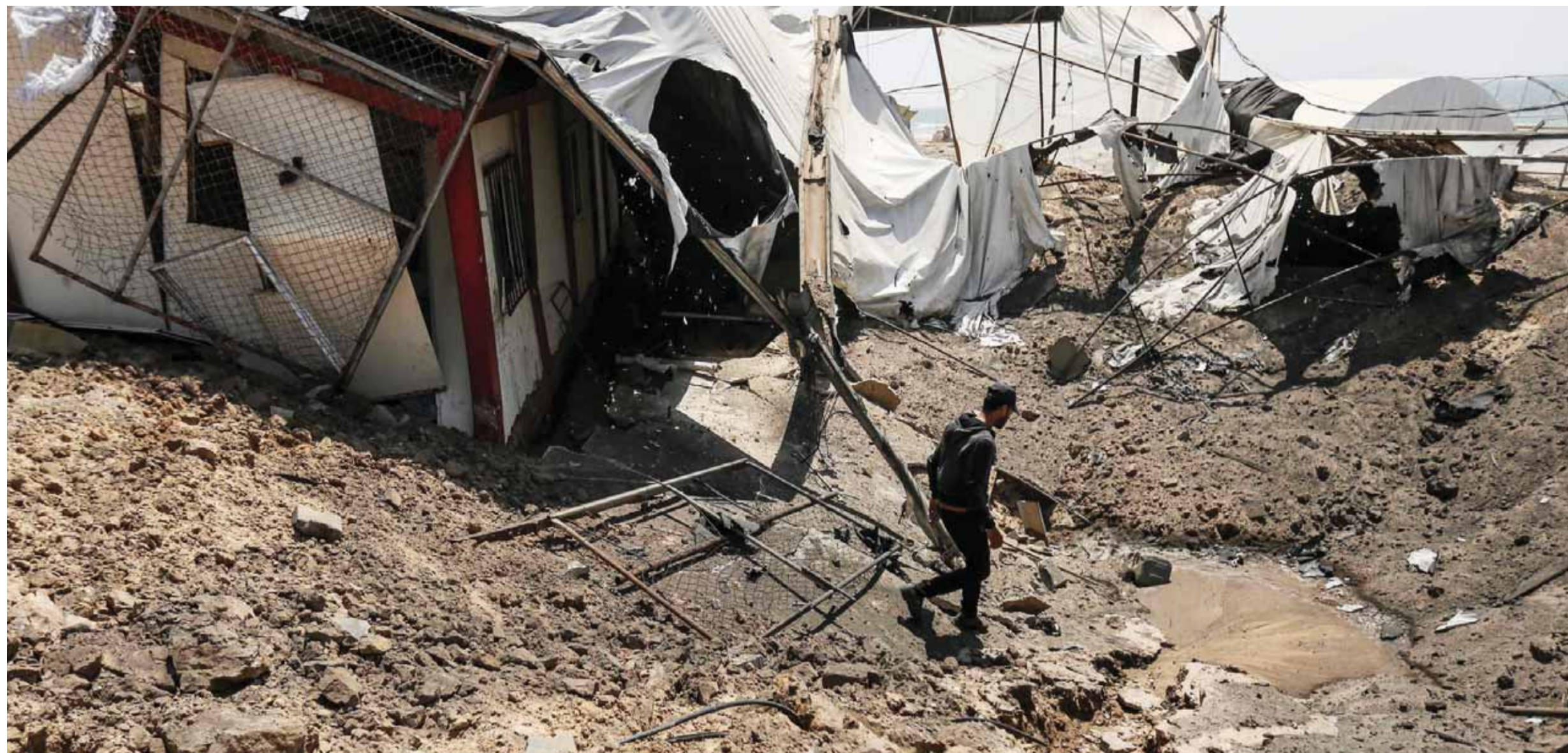
GAZA: A man inspects the damage at a site targeted by an Israeli air strike a day before in Khan Younis in the southern Gaza Strip yesterday. — AFP
