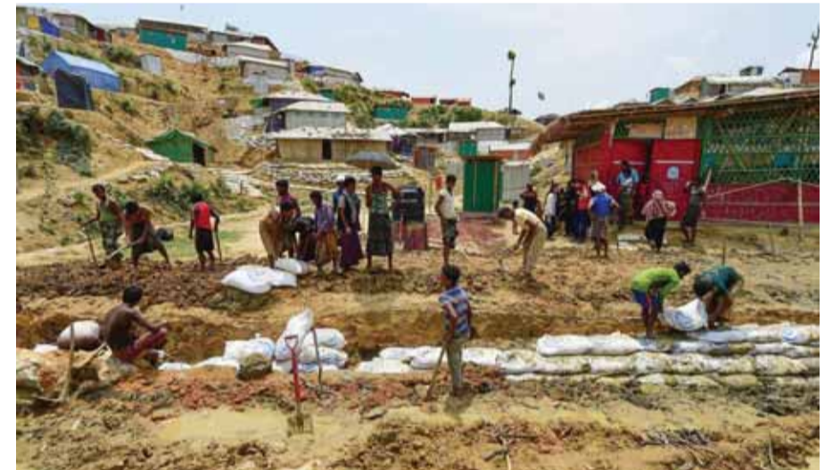
In this photograph taken on May 8, 2018, Rohingya refugees make a drainage canal in preparation for the upcoming monsoon season in the Kutupalong refugee camp in Ukhta. — AFP
