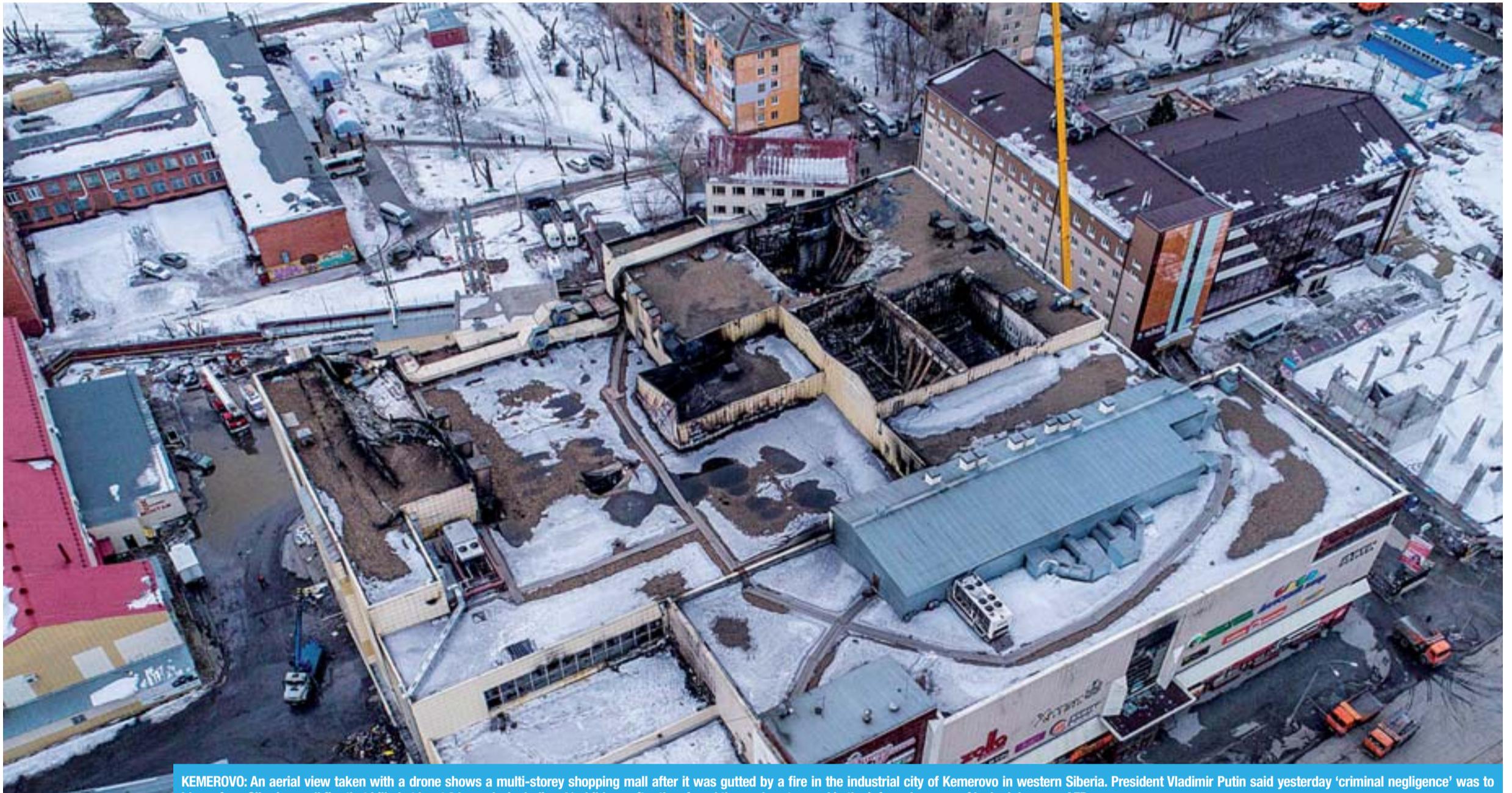
KEMEROVO: An aerial view taken with a drone shows a multi-storey shopping mall after it was gutted by a fire in the industrial city of Kemerovo in western Siberia. President Vladimir Putin said yesterday 'criminal negligence' was to blame for a Siberian mall fire that killed at least 64 people, including 41 children, after they found themselves trapped in the inferno because of locked doors. —AFP
