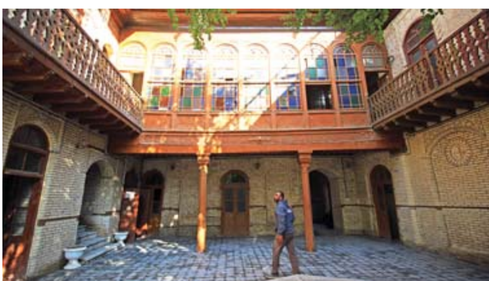
An Iraqi man walks in the courtyard of an old building with traditional 'shanasheel', finely crafted bay windows complete with intricate wooden latticework and ornate stained glass which allow inhabitants to see outside without being seen, in the southern city of Basra. — AFP
