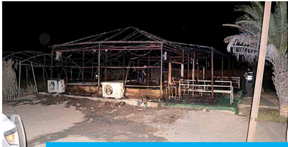
The tent's frame is seen after the fire was extinguished.
