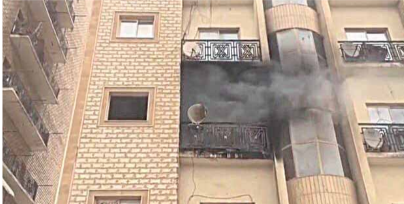
KUWAIT: Smoke is seen coming out from an apartment in a Khaitan building.
