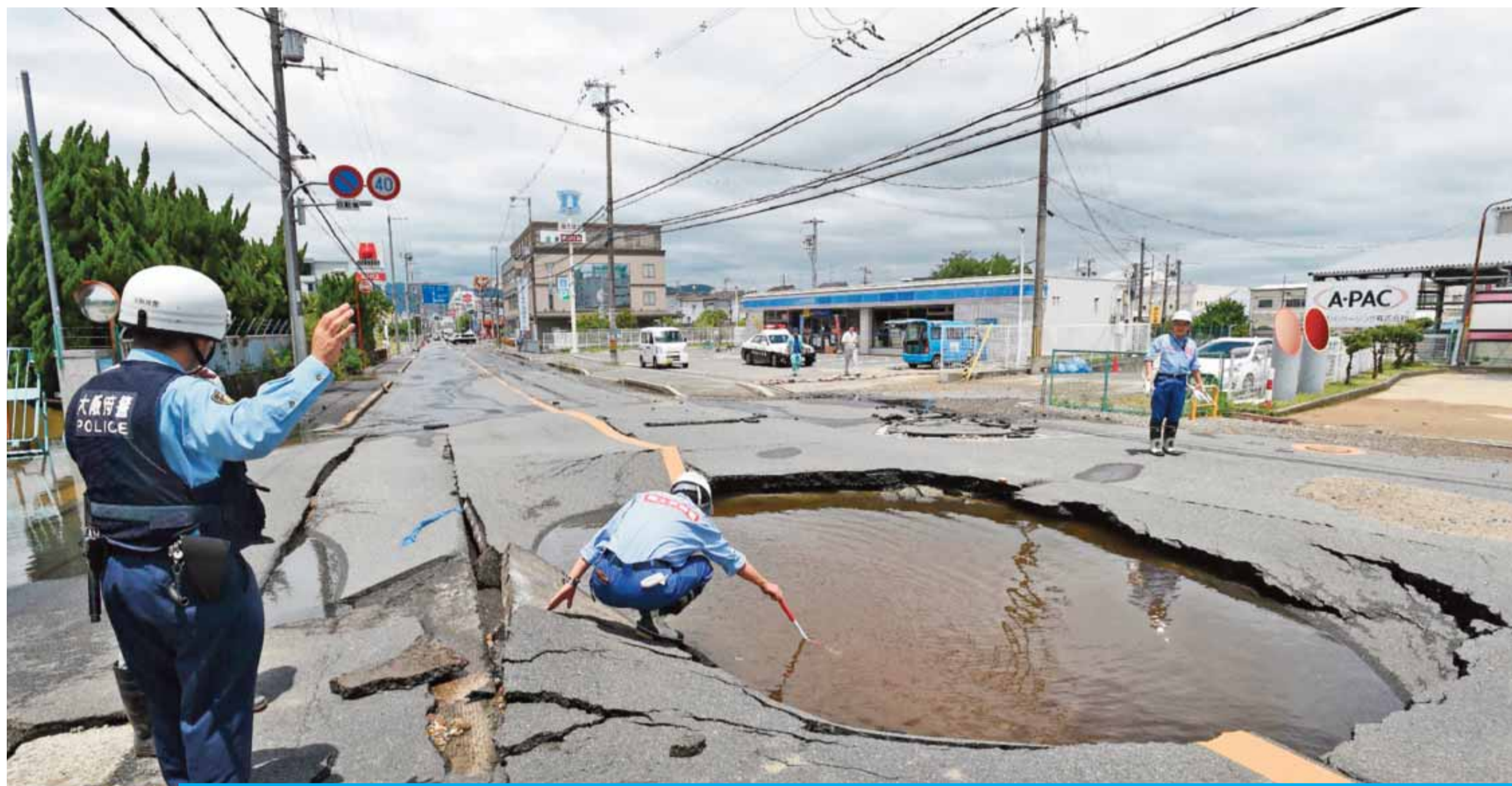
TAKATSUKI: Police check a collapsed road following an earthquake in Takatsuki, north of Osaka prefecture yesterday. — AFP
